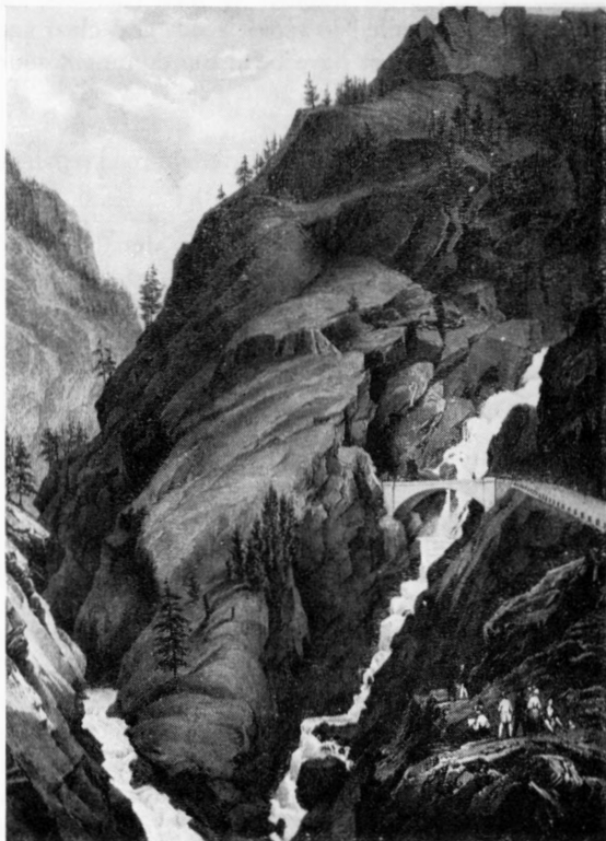
69 Tunnel near Gondo (Simplon Pass)
